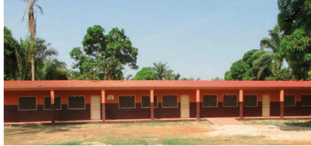
Seven newly constructed classrooms.
