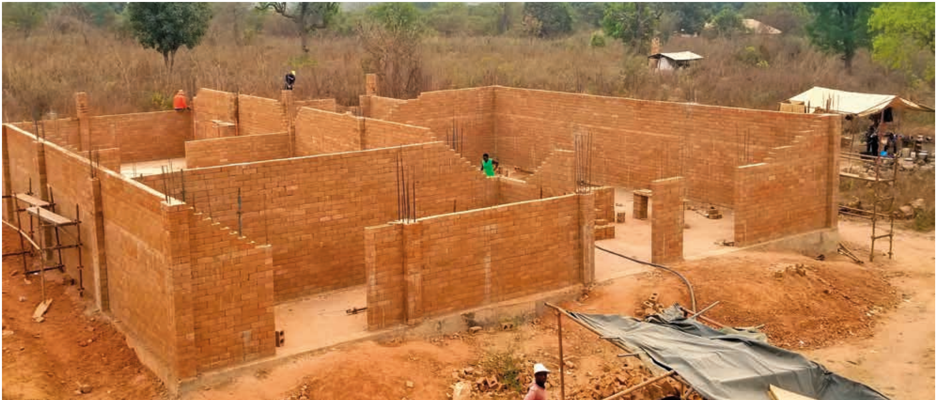
Construction of the Cashew Processing Center.
