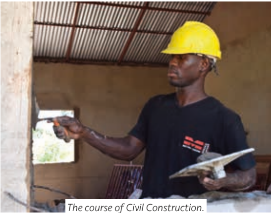
The course of Civil Construction.
